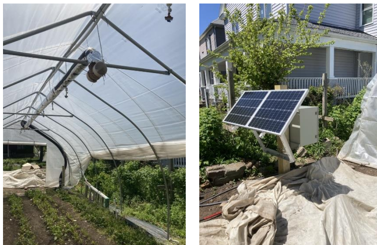
Figure 3 L: EAHX air distribution in tunnel. R: solar panel at site
